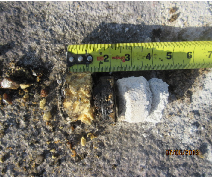
3. ROOF CORE ON AREA "D"
