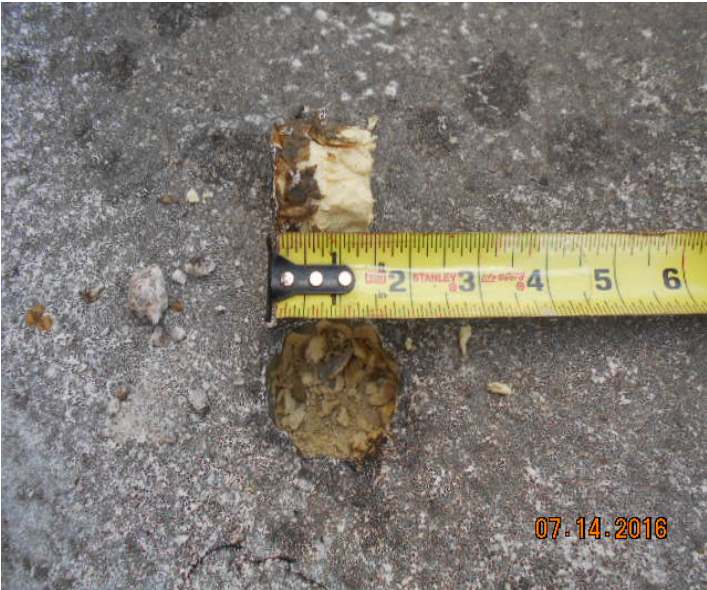
4. ROOF CORE ON AREA "H"
