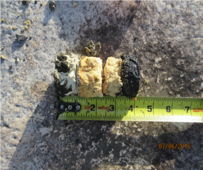
2. ROOF CORE ON AREA "B"
