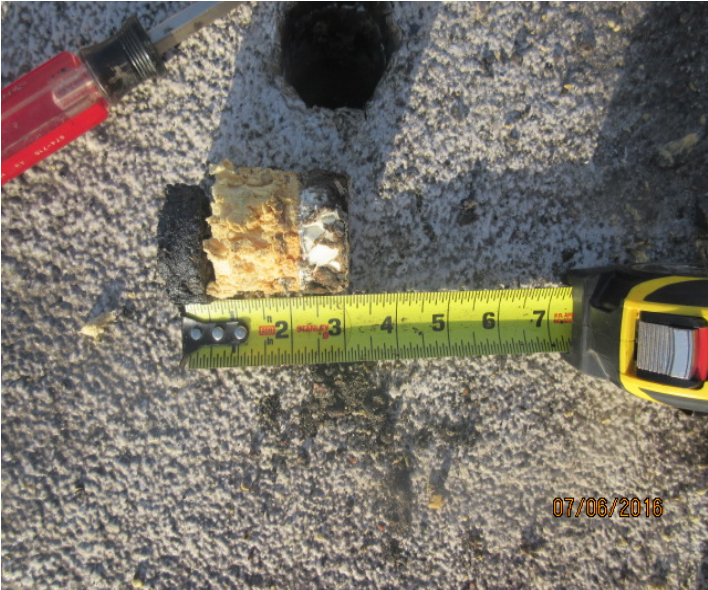
1. ROOF CORE ON AREA "A"
